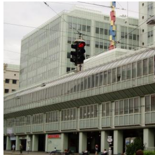
Freihaus building: the conference venue
